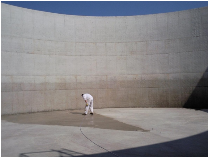
Biogas plant in Germany
