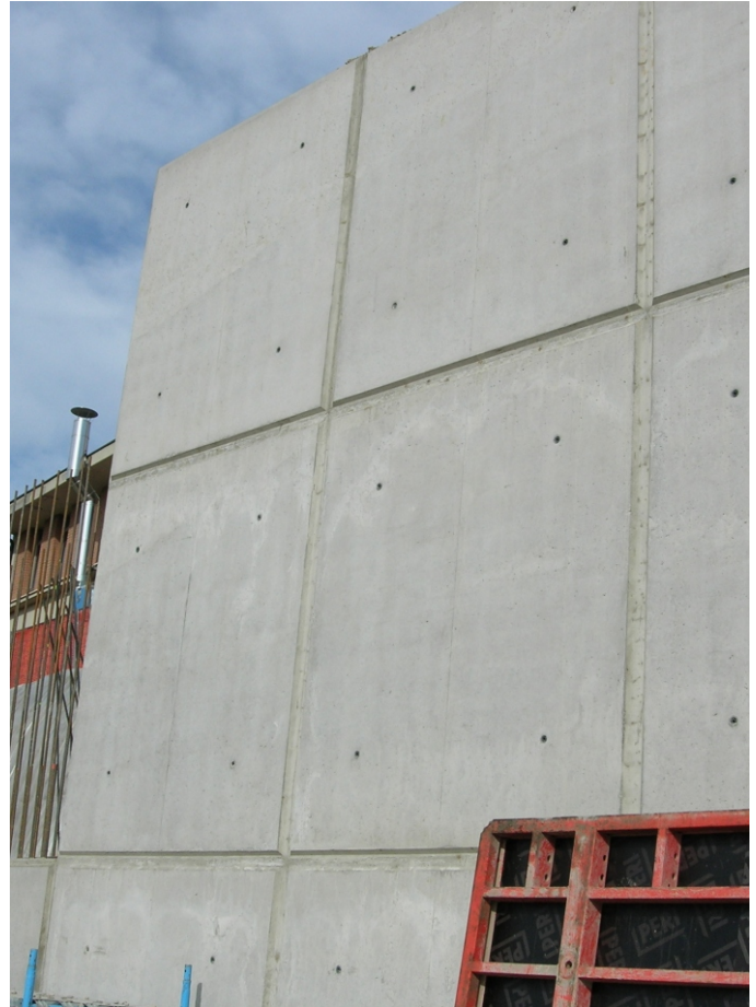
Concrete wall. As it sets concrete diminishes its volume by 1%
