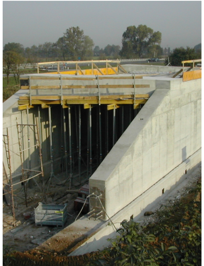
Carugate underpass (Milano, Italy)
