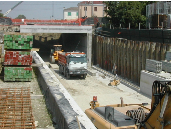
Fontaniva underpass (Padova, Italy)
