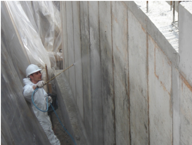
Above ground walls in Castelnovo (Vicenza, Italy)
