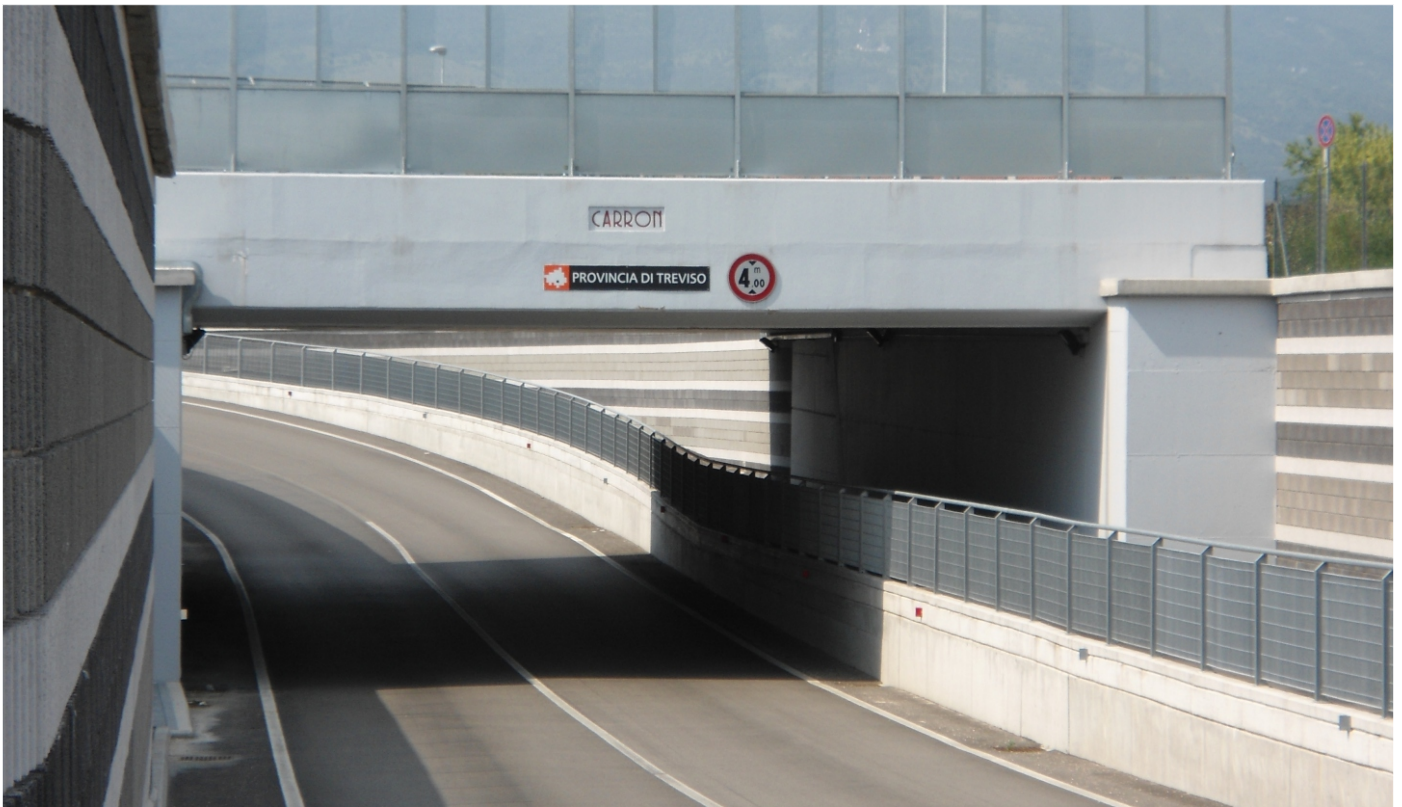
Orsago underpass (Treviso, Italy)
