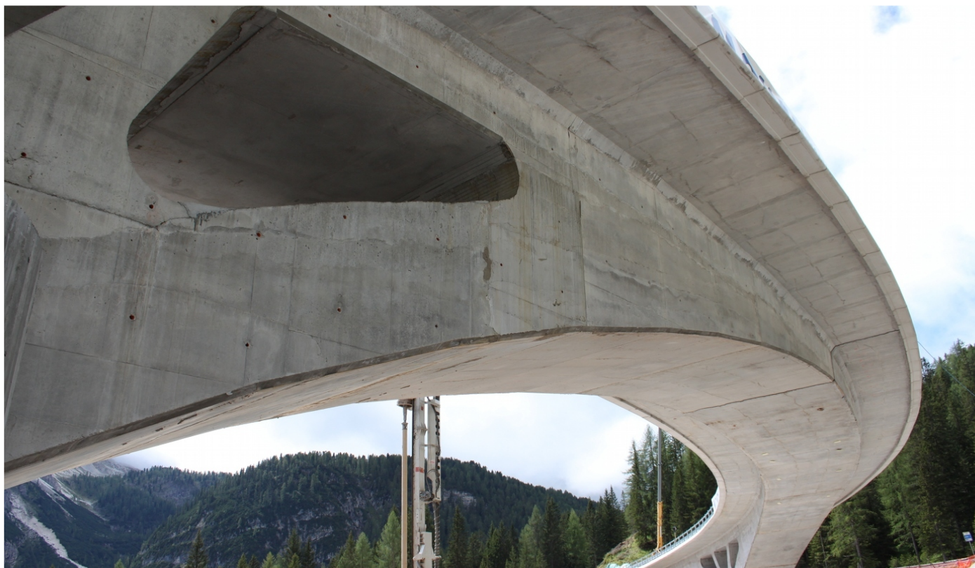
Bridge on Rudavoi stream, Cortina (BL) Italy
